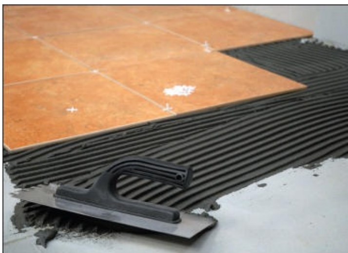
▲ Applying tile glue to the subfloor
