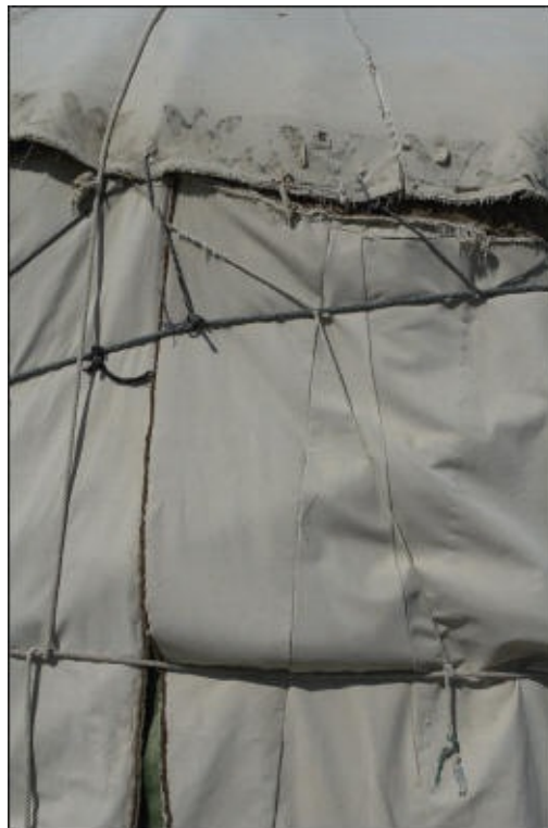
▼ Yurt outer waterproofing fabric
