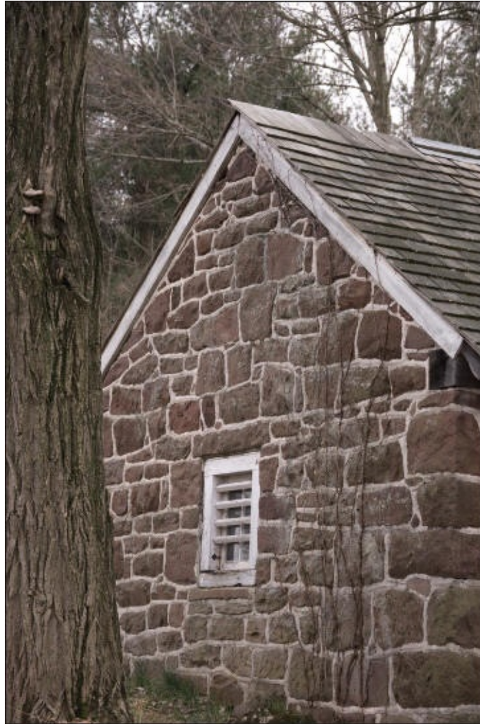
▲ House built with stones shaped with a hammer
