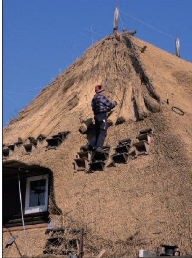
▲ Binding the straw to the roof
