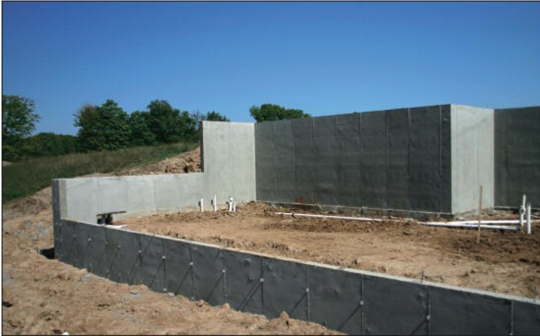
▲ Concrete basement wall and foundation
