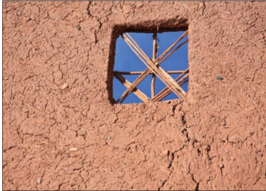
▲ Mud spread over a lattice
